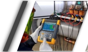
POWER QUALITY ANALYZER
